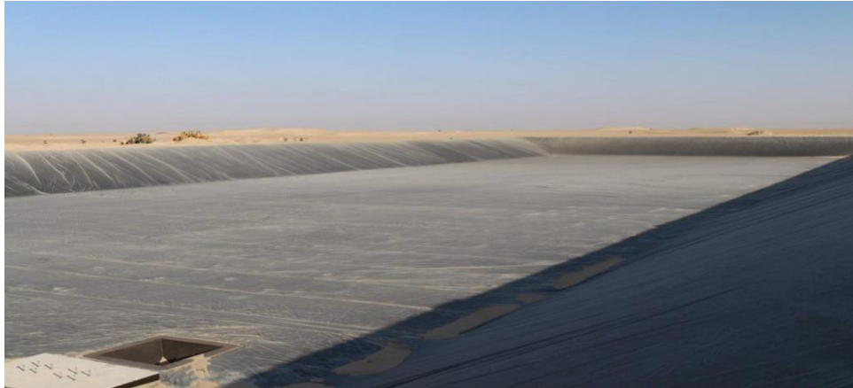
Figure 5. Water drainage system in the Gallo field
